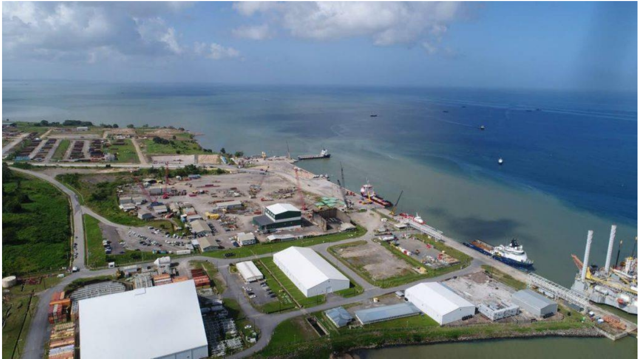
La Brea Industrial Estate and the Port of Brighton. Photo courtesy National Energy Corporation. -
