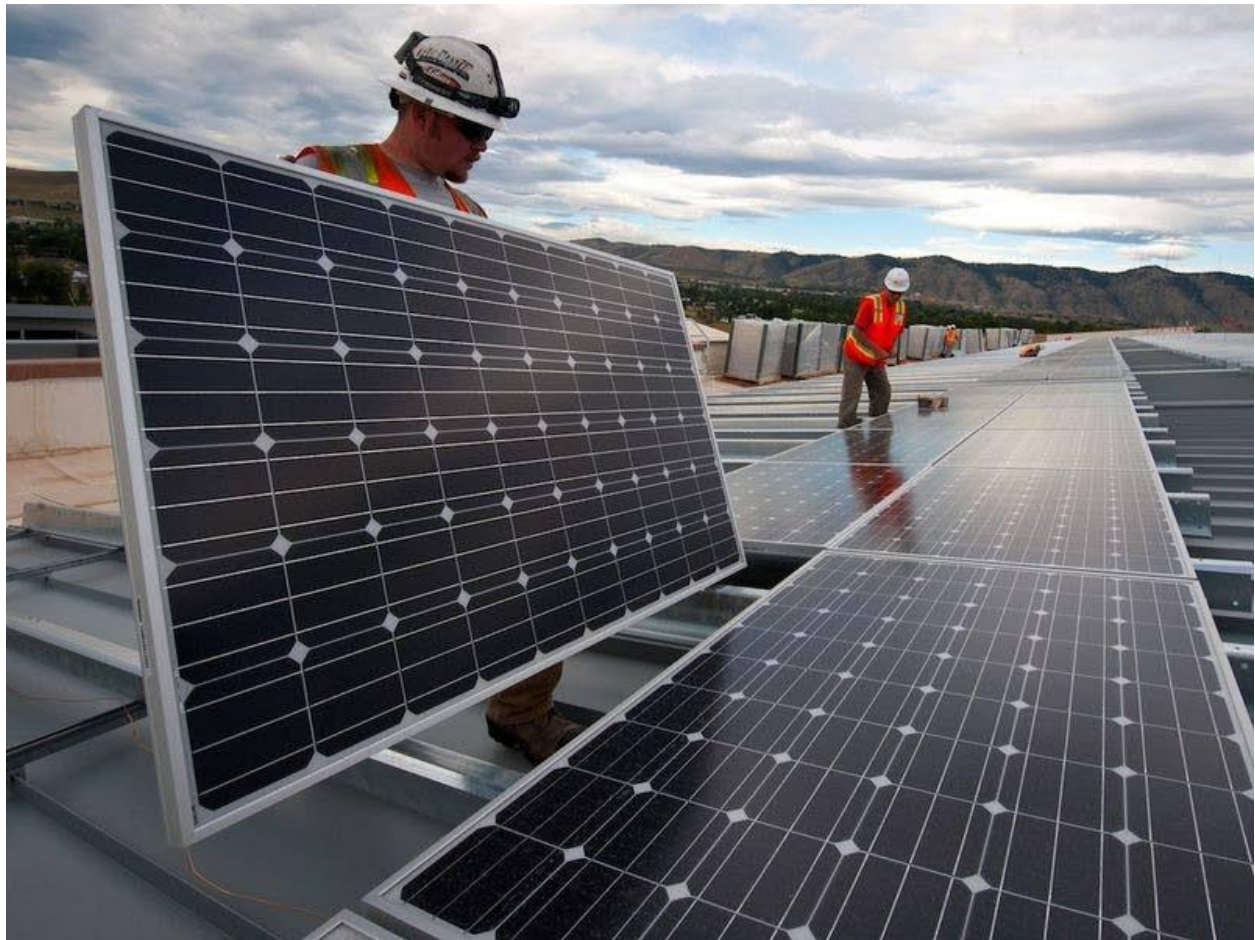
Solar panels being installed.
