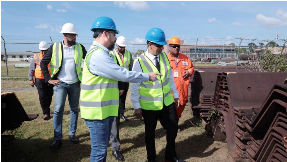
The Honourable Stuart Young, Minister of Energy and Energy Industries, and Senator the Honourable Rohan Sinanan, Minister of Works and Transport, inspect steel sheet piles at National Energy's Couva Storage Facility
