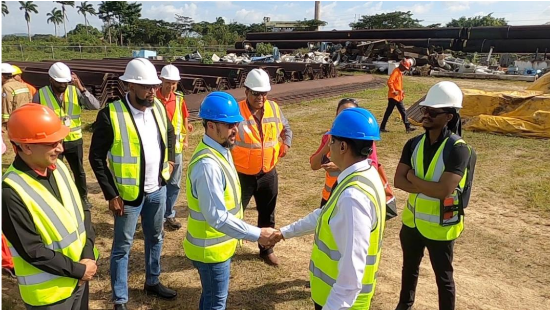
The Honourable Stuart Young, Minister of Energy and Energy Industries, and Senator the Honourable Rohan Sinanan, Minister of Works and Transport, shake hands during a walkabout at National Energy's Couva Storage Facility where 1000 Steel Sheet Piles were officially transferred to the Ministry of Works and Transport. Looking on (from left) are Dr. Vernon Paltoo, President, National Energy and Dr. Joseph Khan, Chairman, National Energy
