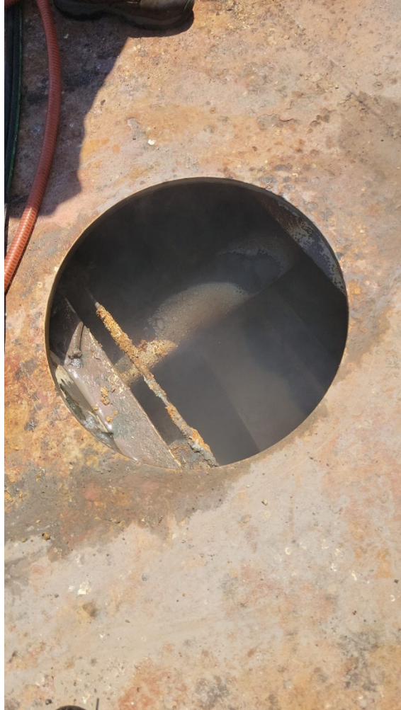
The successful penetration of the first tank.
